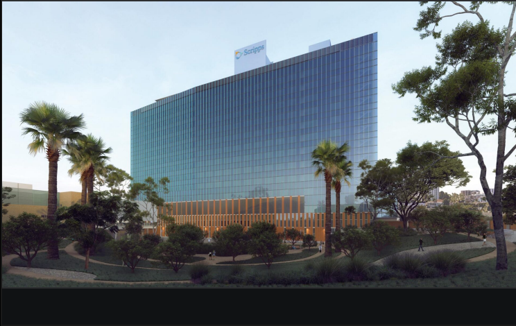
Replacement tower — view
